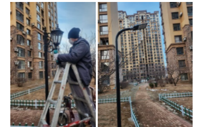
▲ 改造前 Before renovation
