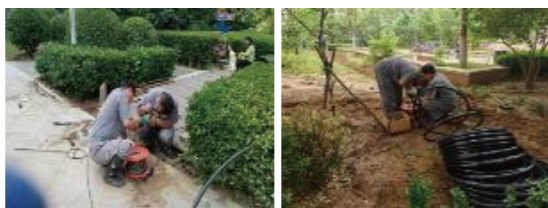
▲ 園區綠化管網改造現場 Retrofitting the landscaping water pipelines
